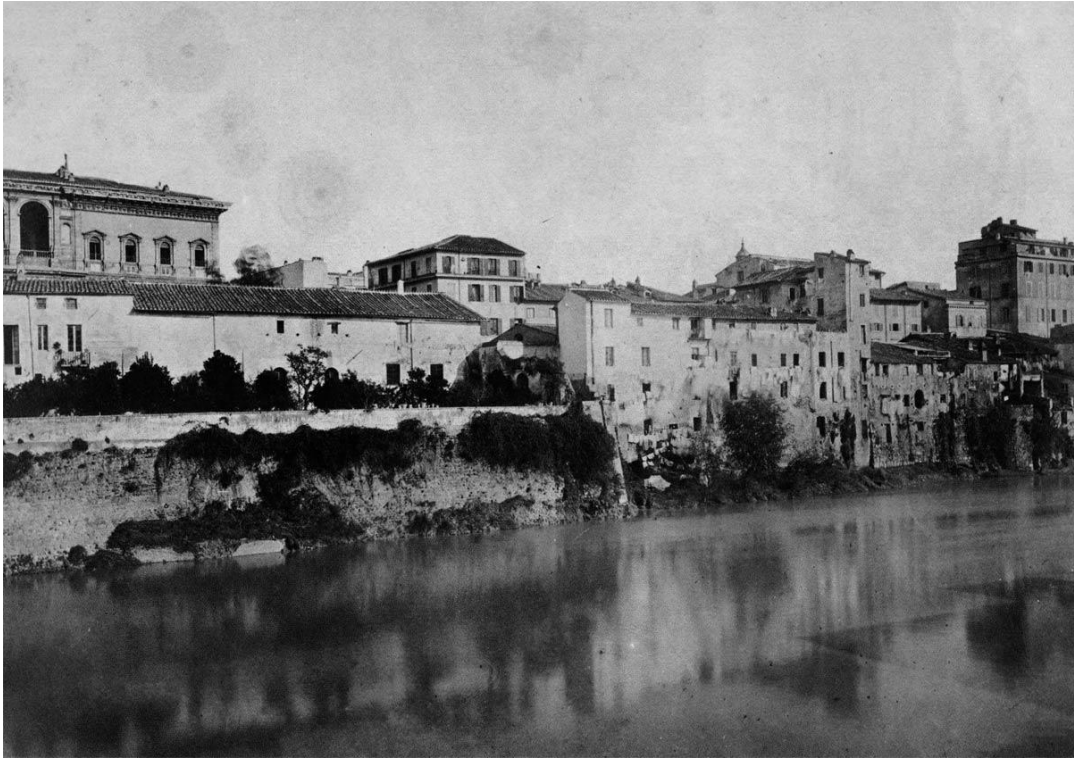
10. Palazzo Farnese (top left) seen from the Tiber before the construction of the river wall (Photo circa 1820)
