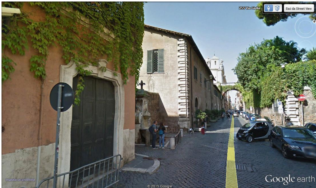
24. View of the existing building from Via Giulia (on the right the Palazzo Farnese garden)
