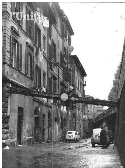
5. The topographical disconnection between the Lungotevere (right) and the older street network in the Tor di Nona area (photo circa 1960)
